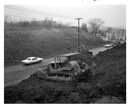
Bulldozer, dump truck and loader on a hilly embankment at a road construction site near Hoosick Street in Troy, NY. Two workmen look on; several cars, buildings, and a Mobil Station are also in view. The image is probably a construction progress photograph, taken by the Dept. of Public Works (related photograph file number 9191).
