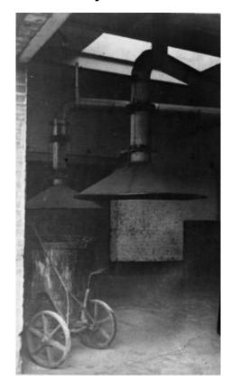
Two fume hoods are suspended from the ceiling, possibly in a laundry facility. A cart in the form of a barrel on wheels rests in the foreground. The image may be described in #32 of "Photographs. 1911" of the "List of Photographs, 1911-1912."
