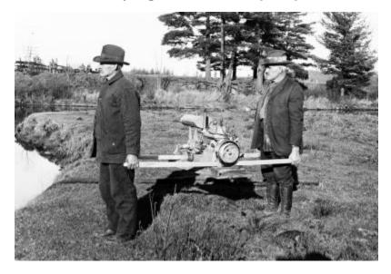
Two Conservation Department rangers demonstrating transportation of a portable Evinrude pump used to supply water to hoses while fighting forest fires. Location unknown, [ca. 1920].
