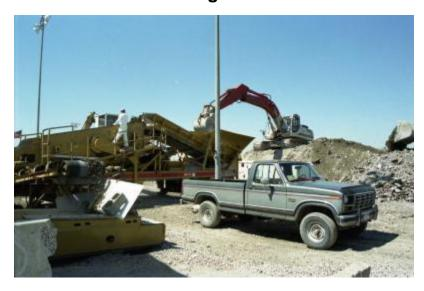
The mound behind the truck that the loader is on is WTC "debris". The material is loaded into a shaker that separates the material by size, then drops onto a conveyor belt. Recovery workers in white suits are doing first inspection as material moves towards shed (left of of photo).
