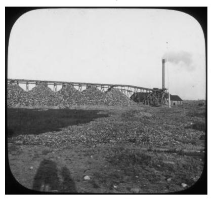
View across the yard of a wood pulp mill, at Au Sable Forks in the Adirondack Mountains. A mill building can be seen with billowing smoke stack and an attached conveyor with large piles of logs nearby.
