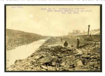
Contract 6. A view of construction looking east from Station 2708 that shows the excavation of a new prism.
