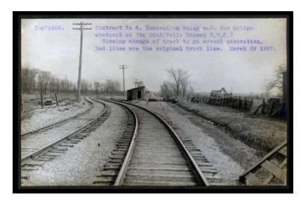
Contract 6. A view of the excavation being made for a bridge abutment at Station 2653 (Falls Branch, N.Y.C.). It also shows the change of the track to go around excavation. The red lines are the original track line.
