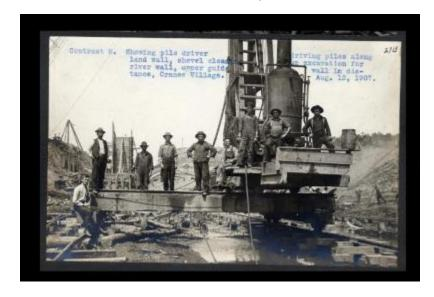
Contract 8. A photograph showing a pile driver driving piles along the land wall, a shovel clearing up the excavation for a river wall, and an upper guide wall in distance in Cranes Village [Cranesville?].
