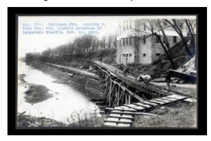
Contract 10. A view looking north from Station 622 that shows progress of the construction of a temporary trestle.
