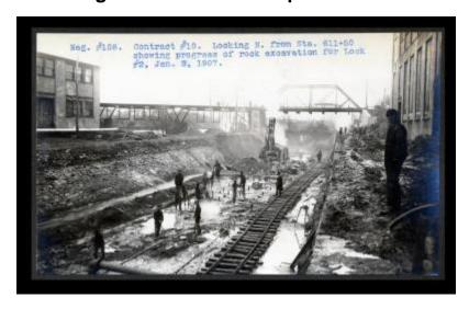
Contract 10. A view looking north from Station 611+50 that shows the progress of rock excavation for Lock 2.
