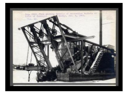
Contract 12. A view showing details of excavation buckets on the front of a conveyor and dredge.
