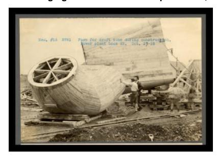
Contract 12. A form for a draft tube during construction of the power plant at Lock 23.
