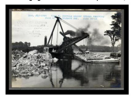
Contract 12. A view north showing a dipper dredge removing rock at the Orchard dam.
