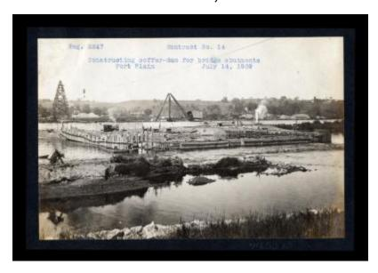
Contract 14. A photo of the construction of a coffer-dam for bridge abutments in Fort Plain.
