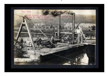
Contract 14. A view showing the dredge at Downing and dredging for the canter-dam in back of lock.
