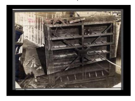
Contract 14. A photo showing the east gates damaged or breaking in the cofferdam at Lock 15 in Fort Plain.
