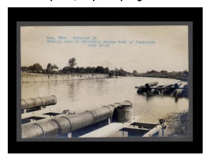
Contract 19. A photo of a channel made by a hydraulic dredge west of Pendleton.
