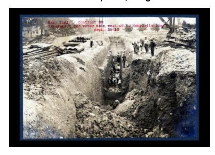
Contract 23. Excavation for water main west of East Henrietta Road. "This photo is looking south; the north half was completed (exc.) on Sept. 14th, and on 15th 72' of 24" C1 Pipe were laid in same. On 16th a cave-in occurred nearly filling the trench; the cave-in is clearly shown here on right side of trench in foreground."
