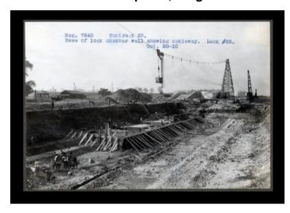
Contract 23. A photo of the base of a lock chamber wall showing cableway at Lock 32.
