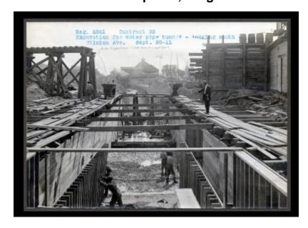
Contract 23. A photo of excavation for a water pipe tunnel looking south at Clinton Ave. (Note Koppel cars & 24" track used here.)
