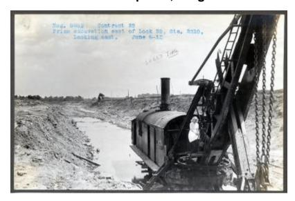
Contract 23. A photo of a prism excavation east of Lock 33 at Station 2210, looking east.
