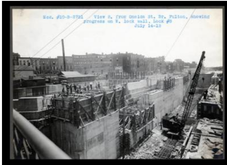
Contract 10B. A view south from Oneida Street Bridge, Fulton, showing the progress on the west lock wall of Lock 3.
