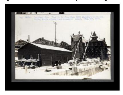
Contract 35. A view southeast from Station 1201 showing storehouse, tools, stone crusher and concrete mixer.
