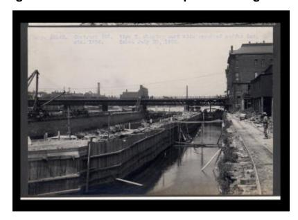
Contract 35. A view north showing the east side of a repaired coffer dam at Station 1204.
