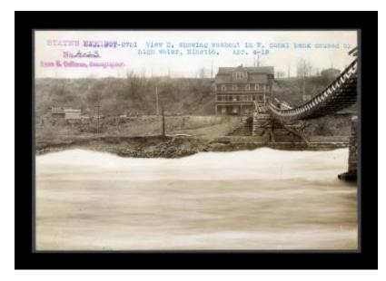
Contract 37. View east showing washout in west canal bank caused by high water, Minetto. State's Exhibit, No. A-23.
