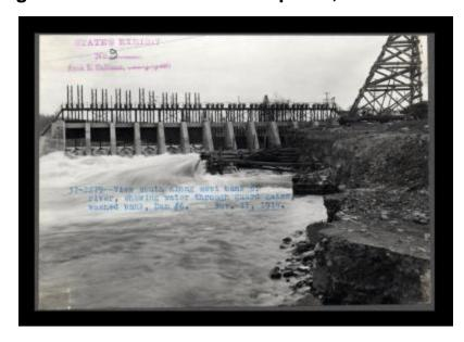
Contract 37. View south along west bank of river, showing water through guard gates, washed bank, Dam 6. State's Exhibit, No. 9.
