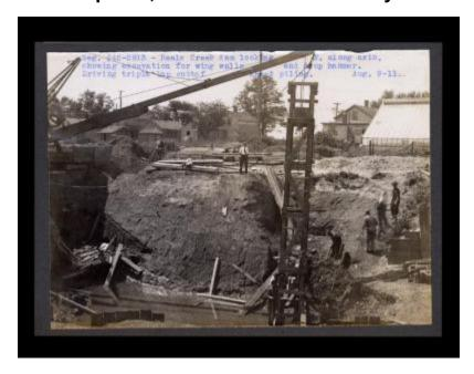
Contract 42. Reals Creek dam looking west along axis, showing excavation for wing walls and drop hammer. Driving triple lap cutoff sheet piling.
