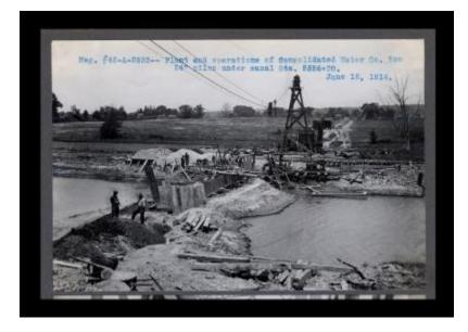
Contract 42A. Plant and operations of Consolidated Water Company, two 24" piles under canal, Station 5556+30.
