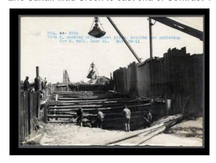
Contract 44. View east showing steel sheet piles, bracing and cofferdam for north wall, Lock 21.
