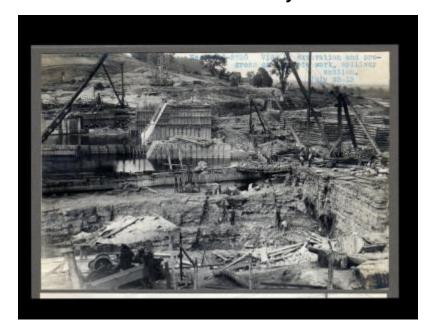
Contract 50. View north, excavation and progress of concrete work, spillway section.
