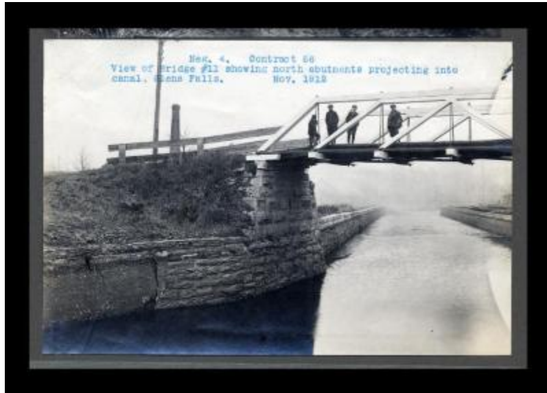
Contract 56. View of Bridge 11 showing north abutments projecting into canal, Glens Falls.
