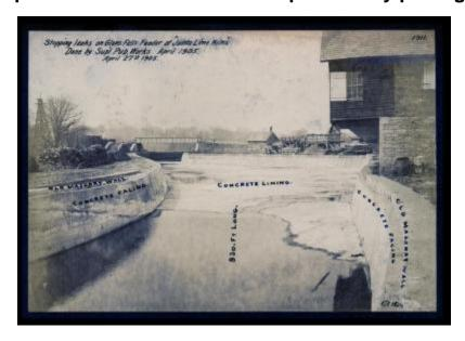
Contract: Miscellaneous Preliminary Champlain Canal - Eastern Divison. Stopping leaks on Glens Falls Feeder at "Jointa Lime Kilns". Done by Superintendent of Public Works, April 1905. HJR Photo.
