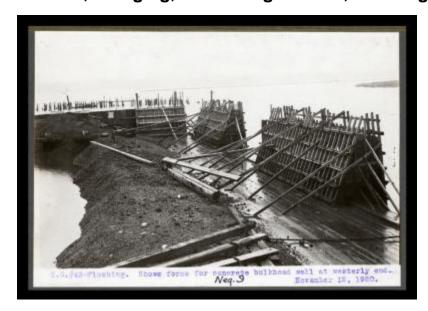
Terminal Contract 43. Flushing. Shows forms for concrete bulkhead wall at westerly end.
