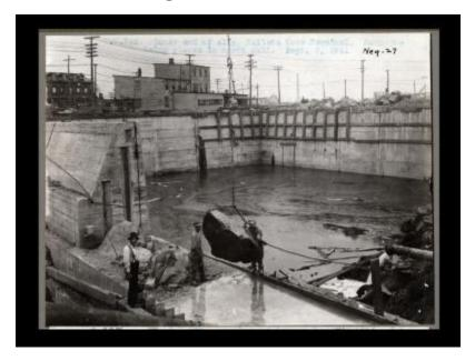
Terminal Contract 45. Inner end of slip, Hallets Cove Terminal. Concrete being placed in north wall.
