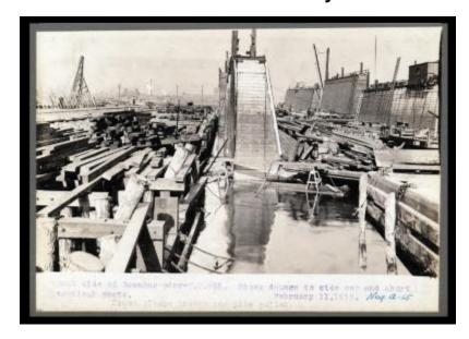
Terminal Contract 55. East side of Gowanus Bay pier--Shows damage to side cap and short vertical posts. Cross clamps broken and pile pulled.
