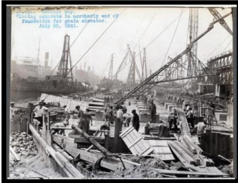
Terminal Contract 81. Gowanus Bay. Placing concrete in northerly end of foundation for grain elevator.
