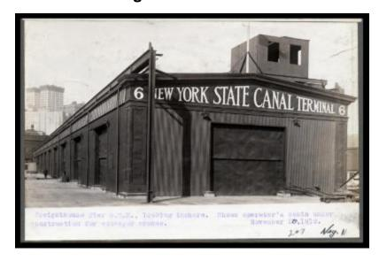
Terminal Contract 207. Freight house Pier 6, E.R. [East River?], looking inshore. Shows operator's cabin under construction for conveyor cranes.
