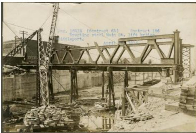
Contract 106. Erecting Steel, Main Street Lift Bridge, Middleport.
