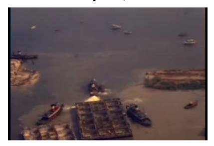
Aerial footage of tugboats moving giant caissons – a type of sophisticated bridge support – for the soon-to-be-built Tappan Zee Bridge.
