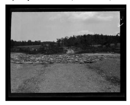
This layer of stone is the overflow spillway built for the expanded Palmer Pond by the Civilian Conservation Corps. Stones used in this fashion to prevent erosion are called "rip-rap." CCC camp S-92, stationed in Almond, has been damming and expanding the pond for recreational use. This image was created to record the reforestation work of the Civilian Conservation Corps under the supervision of the New York State Conservation Department.
