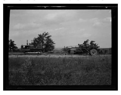
A tractor and a grader for the rough truck trails built by the Civilian Conservation Corps sit on a work in progress. This trail was likely constructed to improve access to a reforestation area and to assist with firefighting efforts. This trail, #202-1, is the work of CCC camp S-123, stationed in Beaver Dams, N.Y. This image was created to record the reforestation work of the Civilian Conservation Corps under the supervision of the New York State Conservation Department.
