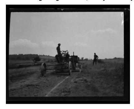
Two of the "boys" from the Civilian Conservation Corps use a tractor and a grader to make a rough truck trail. This trail is likely being constructed to improve access to a reforestation area and to assist with firefighting efforts. This trail, #202-1, is the work of CCC camp S-123, stationed in Beaver Dams, N.Y. This image was created to record the reforestation work of the Civilian Conservation Corps under the supervision of the New York State Conservation Department.
