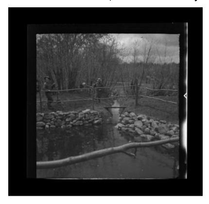
Workers from the Civilian Conservation Corps, camp S-134, have finished a waterhole to aid fire suppression. The hole has been excavated, lined with stone and connected to the nearby brook to provide a source of water to fire fighters. Camp S-134 is stationed in Canton, N.Y. This image was created to record the reforestation work of the Civilian Conservation Corps under the supervision of the New York State Conservation Department. The photograph was taken by John Clawson, foreman of the camp.
