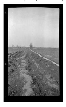
A fire break has been gouged into the ground in this empty field by the Civilian Conservation Corps, camp S-125, stationed in Slaterville Springs. The gap in the vegetation will hopefully stop the spread of a grass fire. This image was created to record the reforestation work of the Civilian Conservation Corps under the supervision of the New York State Conservation Department.
