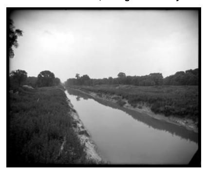
View of "Dead Man's Bend," somewhere in Livingston County. View shows the condition of an old channel opposite cut off number 7. The channel is narrow and winding, with dead trees falling in and growth on the banks that impede stream flow.; The purpose of this image is unknown.
