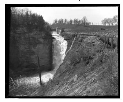
View of a dam on the Deer River at Copenhagen in Denmark, Lewis County. A penstock line is running to a powerhouse of the Deer River Power Corporation. The exposed bedrock is shale and siltstone dating from the Ordovician Period (the span of the Earth's history from about 505 to 438 million years ago.). This image was created to record the waterpower activities of the New York State Conservation Commission.
