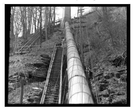
View of a penstock (gate for controlling water flow) and the lower end of a standpipe (vertical pipe into which water is pumped to produce a desired pressure) at the plant of the Deer River Power Corporation at Copenhagen in Denmark, Lewis County. The total head is 165 feet. This image was created to record the waterpower activities of the New York State Conservation Commission.
