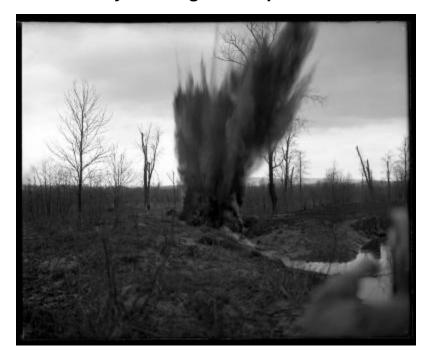
View of a dynamite explosion in action. The dynamite was exploded in a ditch on farmland. The purpose of the work was to improve drainage. This photograph depicts field work of the Conservation Dept.
