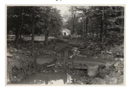
Trenches dug during the construction of a pond at the State operated Summitville Fish Hatchery in the Catskill Mountains. One building and several men are visible.
