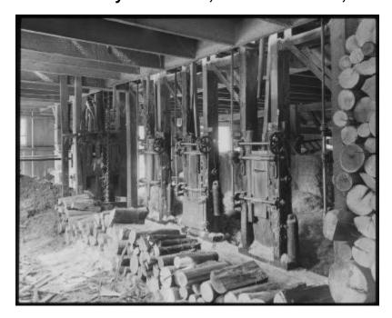
Interior view of an excelsior factory at Phoenicia in the Catskill Mountains. Included in view are blocks of wood, machines and bales of excelsior, which is a trade name for short, thin, curled shavings of soft wood used for stuffing cushions and mattresses.
